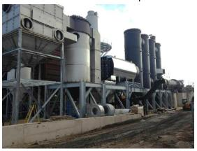
Work continues with the new oxidiser. It was also discussed that this will improve the energy consumption on site by burning biomass instead of fossil fuels (reducing carbon emissions) and by generating electricity via a steam turbine.
