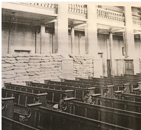
Figure 3 Sandbags in Drill Hall
