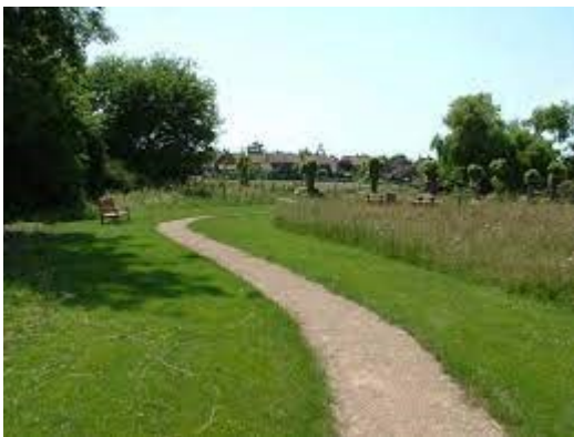
Fig 6. Path images (hardcore 150mm, 20-30mm gravel dusting, 2metre wide)
