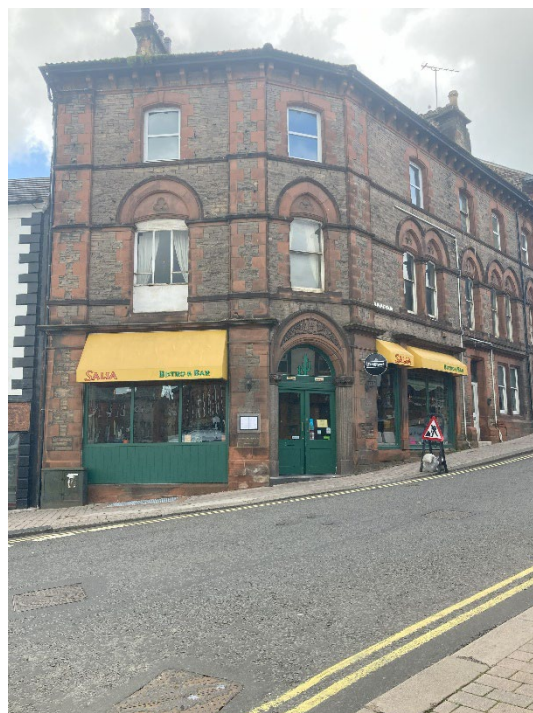
Figure 17 String courses and brackets to eaves on building in Castlegate
