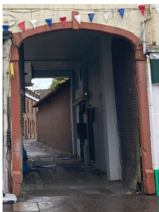
Figure 13 Example carriage doorway
