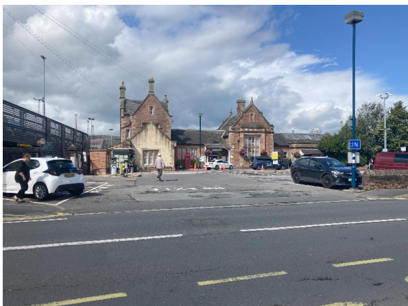
Figure 49 Penrith train station
